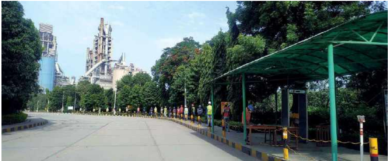
The Narsingarh Plant: pedestrian walkway.
