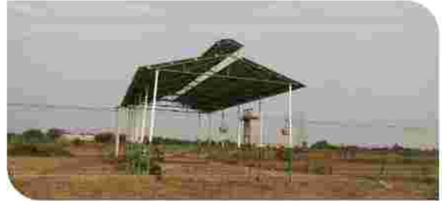
Road & shed Construction
