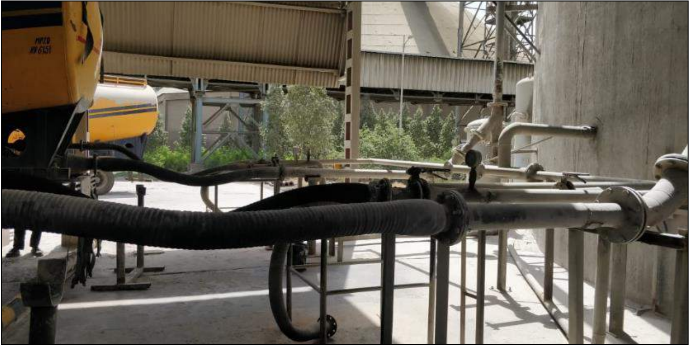
Annexure-9: Pneumatic Fly Ash Unloading
