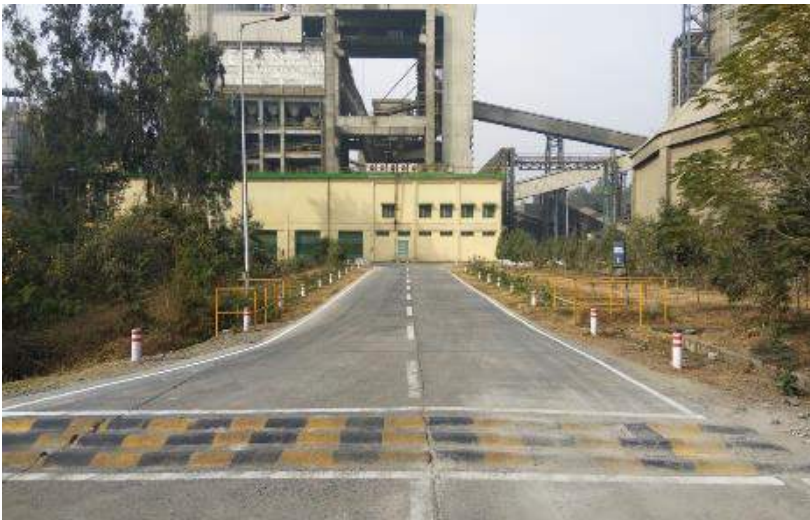
Annexure-10 : Concreted Road Inside Plant
