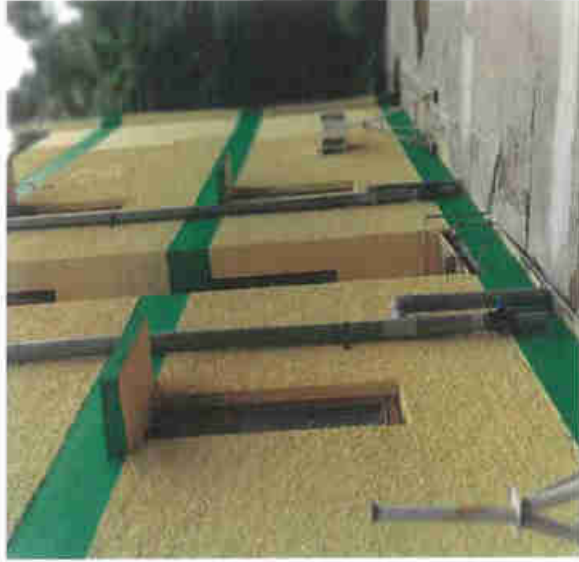
Pipe Lines Laying
