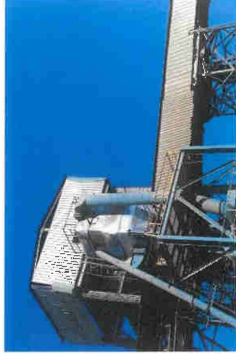
Installed Big Filters at Fly Ash Silo
